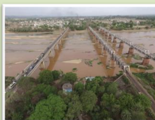
Road/ Rail Over Bridge, Brahmani River, Panposh
