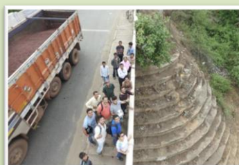
Road Over Bridge at Panposh
